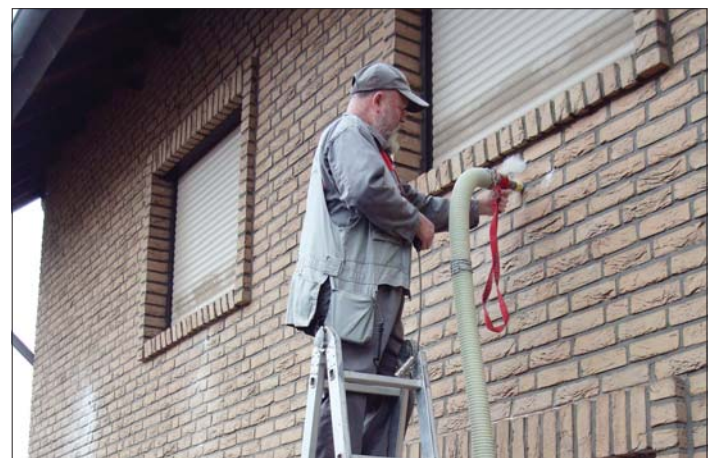
Cavity wall insulation
