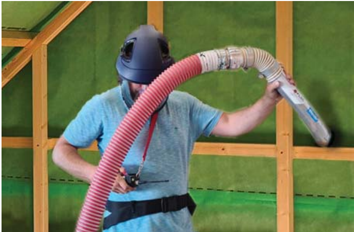
Rotary hose connectors (SDV) facilitate working with the injection needle
