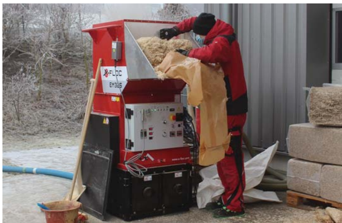
Filling the machine with the natural insulation material
